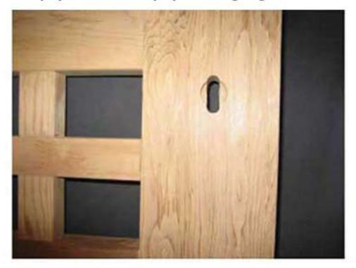
The #40-300 Thumb Latch arrives with a 1" dia bore recessed 3/8".
